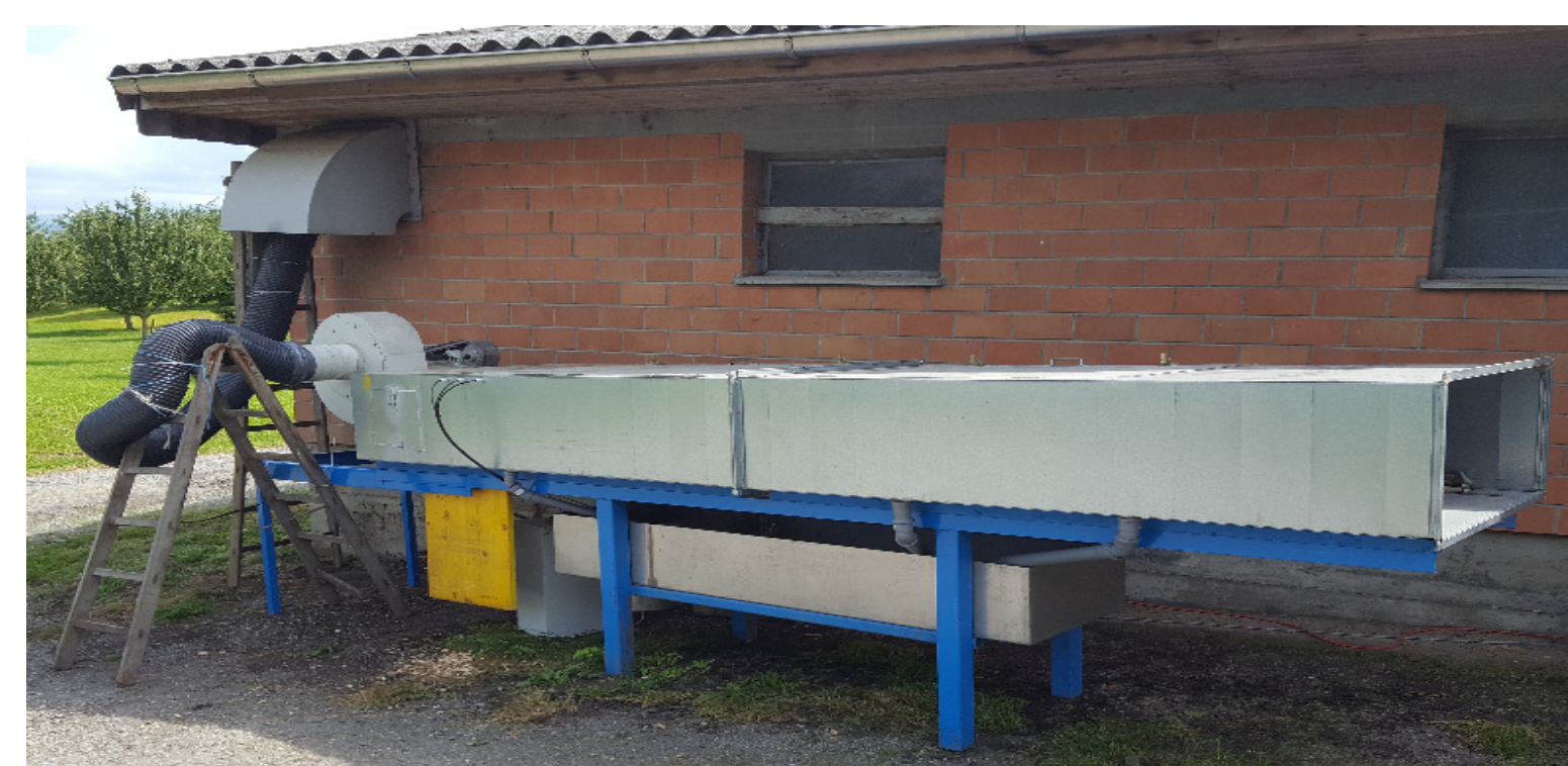
BABS 1m 3 filter connected on extracting air of a poultry farm
